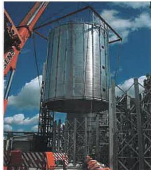
Hopper being lifted externally off the hip section, prior to any hopper panels being fitted.
