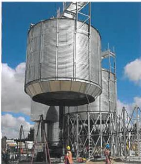
Hopper being lifted into position from inside the silo, brackets attached to hip section.
